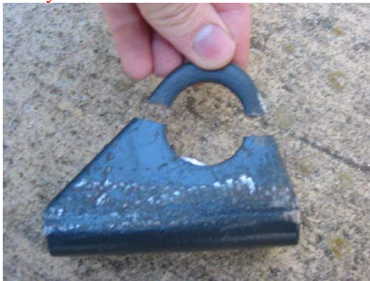
Fig 4 Two small cuts on the new bracket that can help in removal of the cylinder you are trying to save in order to replace it in the original bracket that is still attached to the frame. Do not make these cuts on the original bracket and do not cut into the cylinder.
